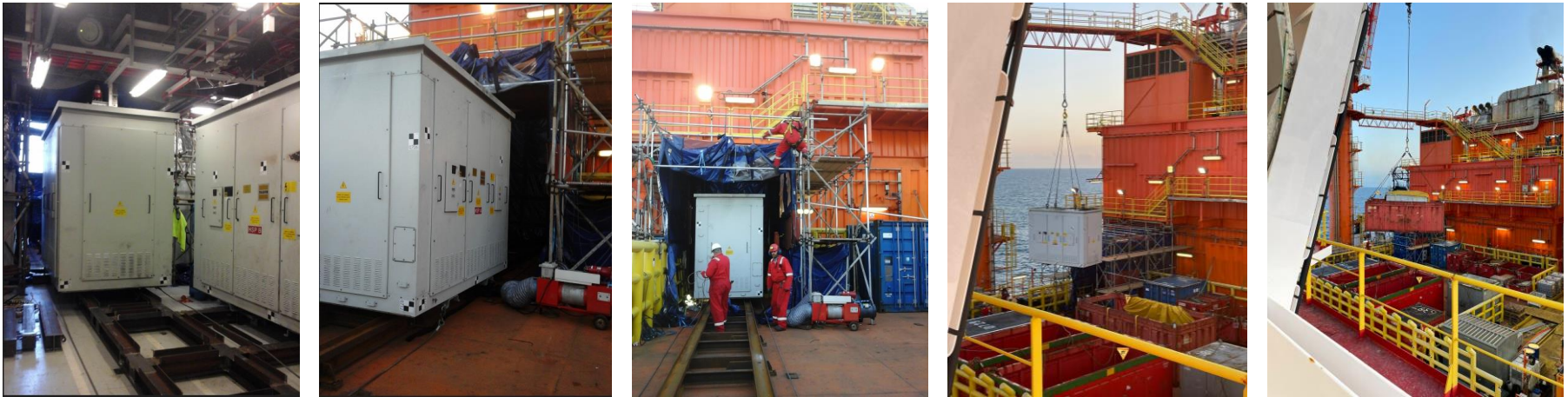
Armada Kraken (L-R): HSP transformers being removed from Kraken to be refurbished. Each of the HSP transformers weighs approximately 16 tons.
