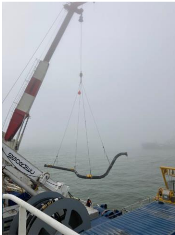
Armada Constructor: Spool installation, Pre-commissioning of pipeline, and demobilization of Armada Constructor
